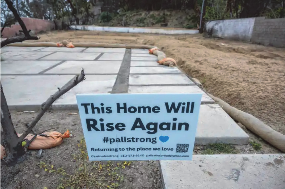
A home destroyed by the Palisades Fire in Pacific Palisades, L.A.
